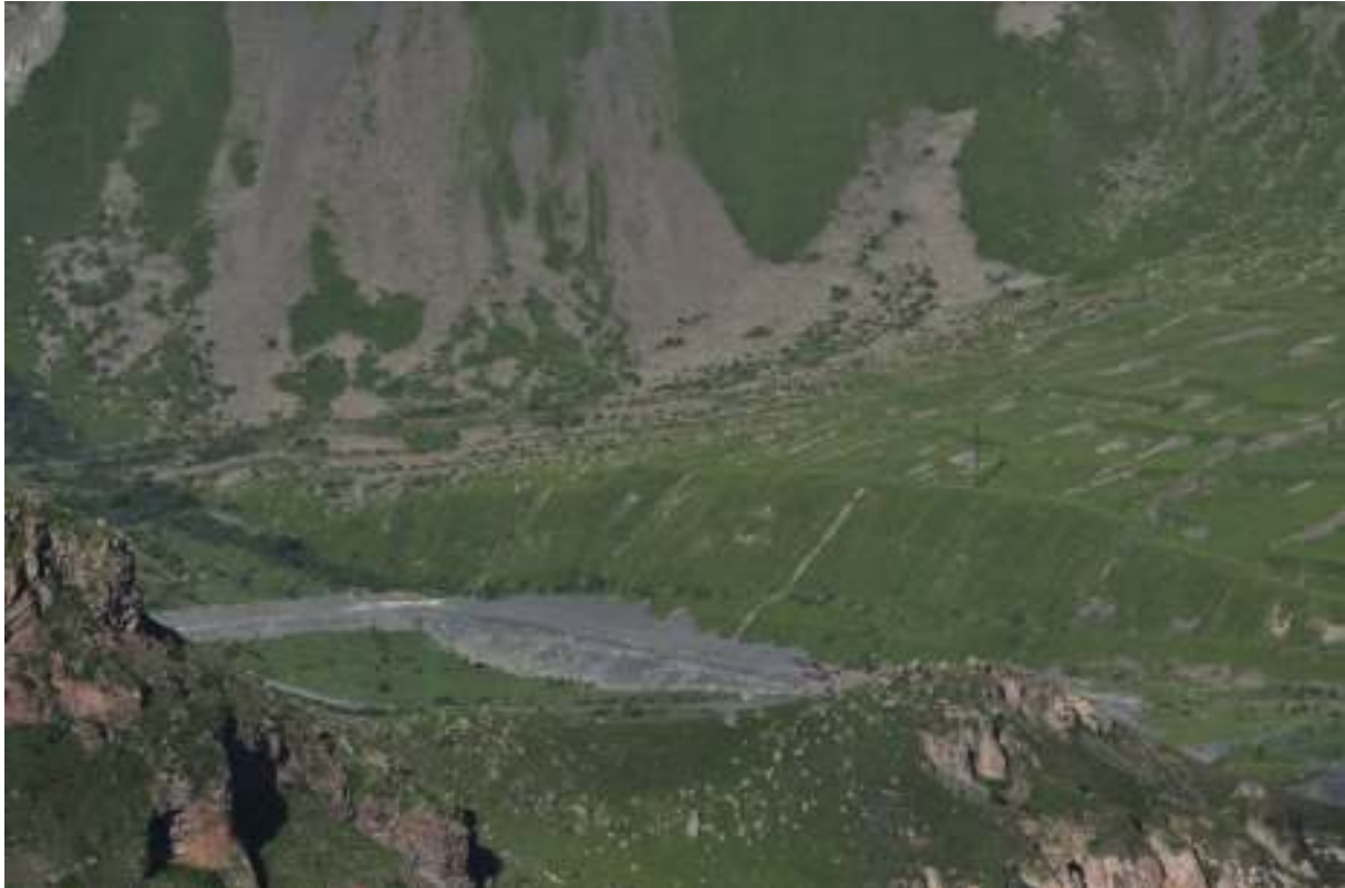
Figure 6: View at the area related to map polygon 153/1 from above, it shows the open erosion areas there even better. Also the course of the power plant line becomes very well visible from this perspective.
