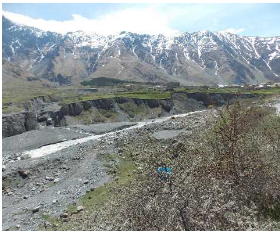
Picture 3.1.1.1. View of dam location area
