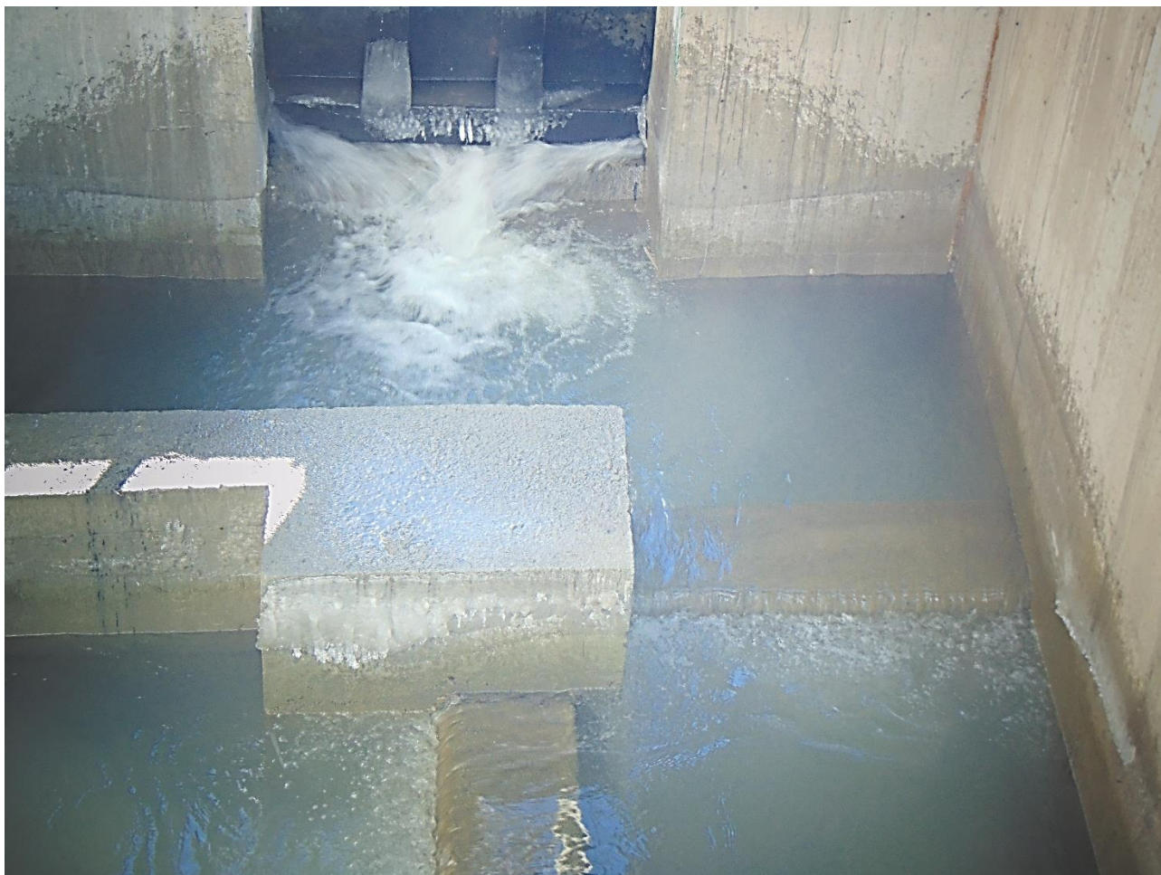
Figure 32. Water leaking during the full closure of the fish pass
