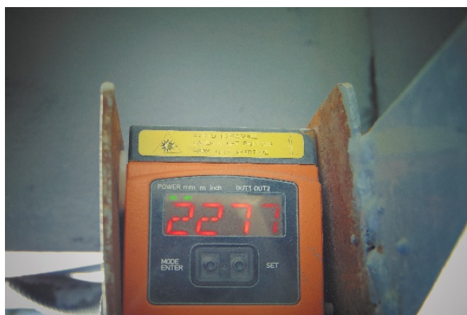
Figure 36. The electronic device showing the level of the openness of the sluice
