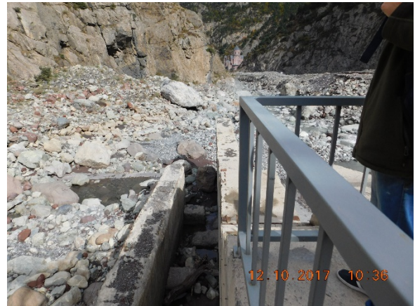
Figure 15. State of the fish pass at Larsi HPP
