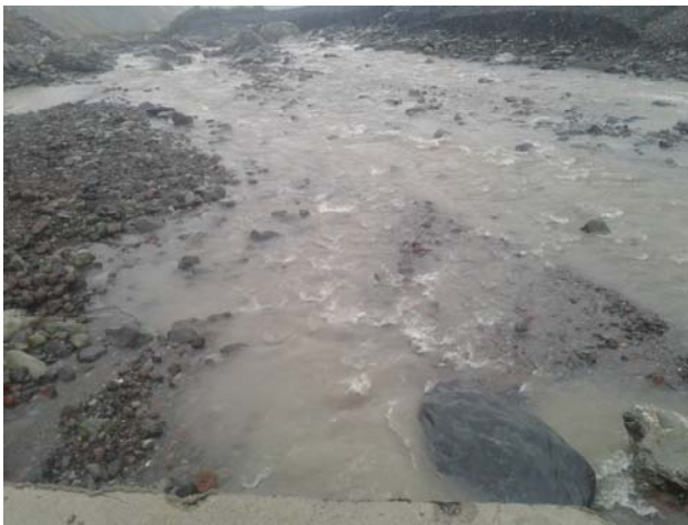
Figure 10. Deepening of the entrance for fish in the lower reach of the fish pass
