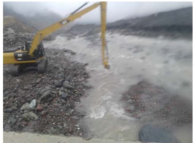
Figure 10. Deepening of the entrance for fish in the lower reach of the fish pass
